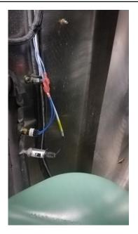
High Pressure and low pressure switches are located in the compressor compartment. The high pressure switch (left picture) must be physically reset if pressure exceeds 600psi. The low pressure switch (right picture) will reset automatically when pressure is above 80psi.
